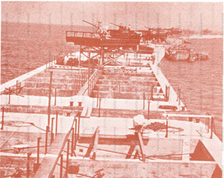
Construction of concrete caisson nearing completion in the London docks. Blockships were scuttled to form part of the northern and seaward breakwaters.
