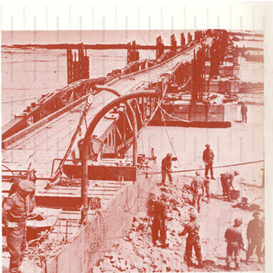
The shore end of a floating roadway at low tide.
